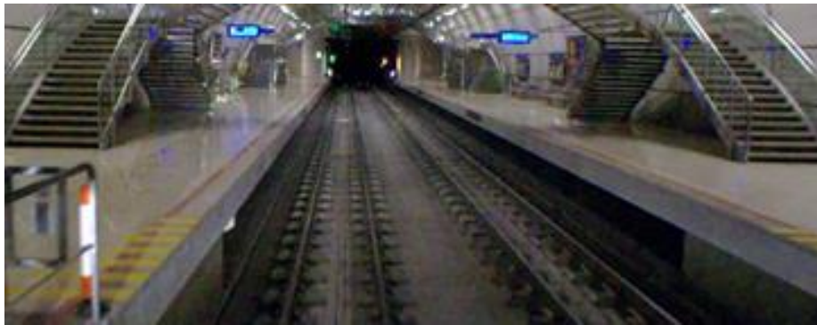
Figure 14 - Platform of the station marked with a red line.
