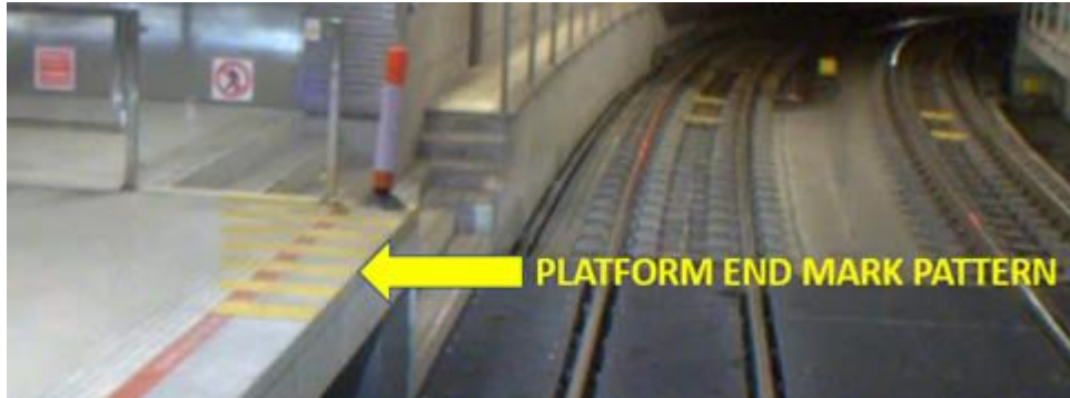
Figure 12 - Platform End Mark Pattern.
