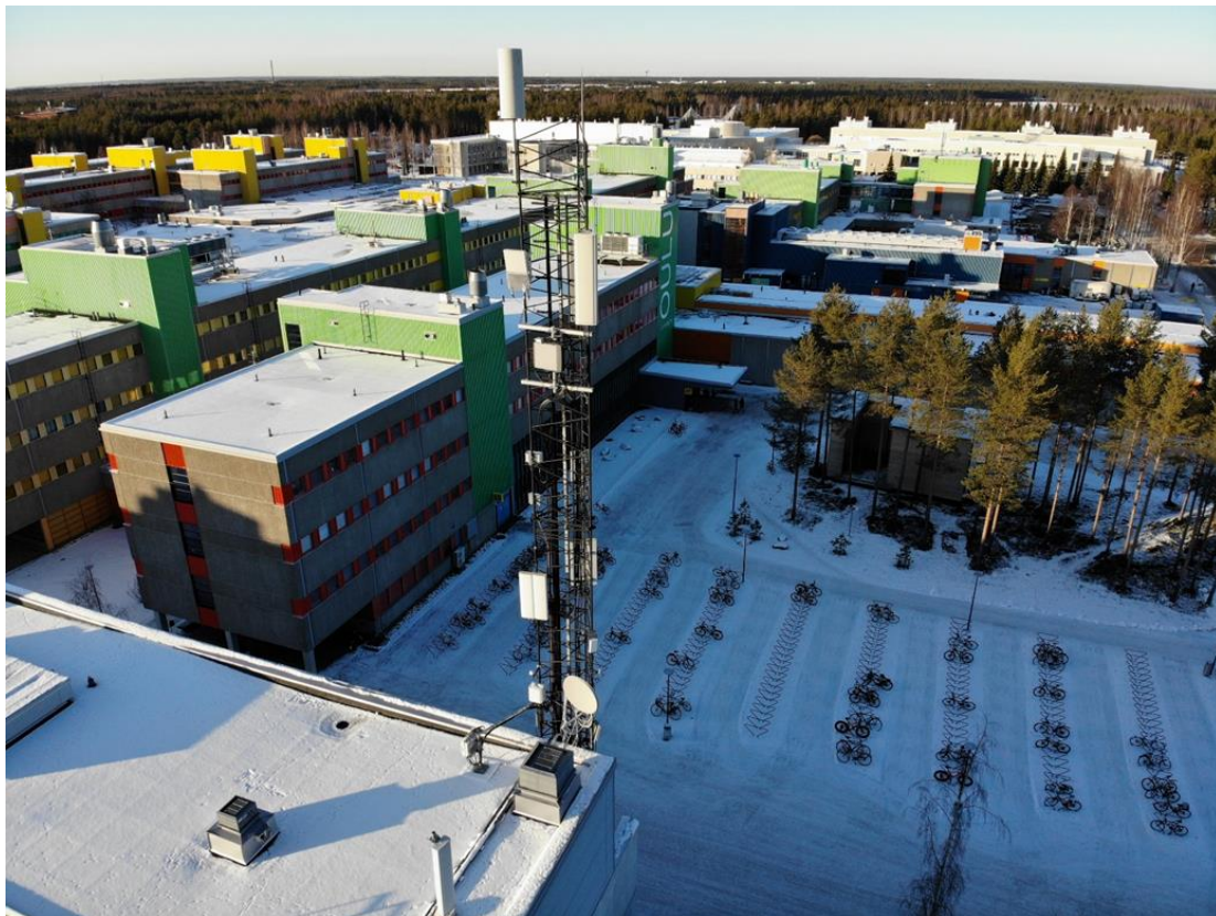
Figure 22 – Antenna tower of the University of Oulu hosting the 5GTN base station’s antenna used in the tests.
